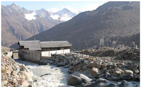
**Figure 1:** Gauging station "Vernagtbach" at 2640 m a.s.l. with the wooden walls to protect the station from high flows, with the climate station on the right. (Photo taken 30 September 2003 by L. Braun).
